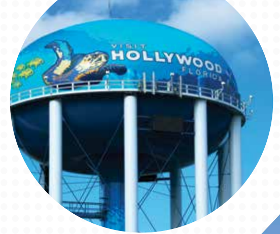
right: 2011 Tnemec Tank of the Year Hollywood, FL
